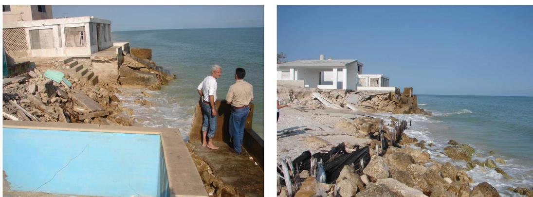
Figure 1. Example of severe beach erosion and property loss in the Northern Yucatán Coast.
